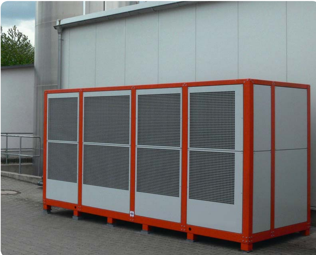
Compact chillers model weco 300 AZ for outdoor installation
